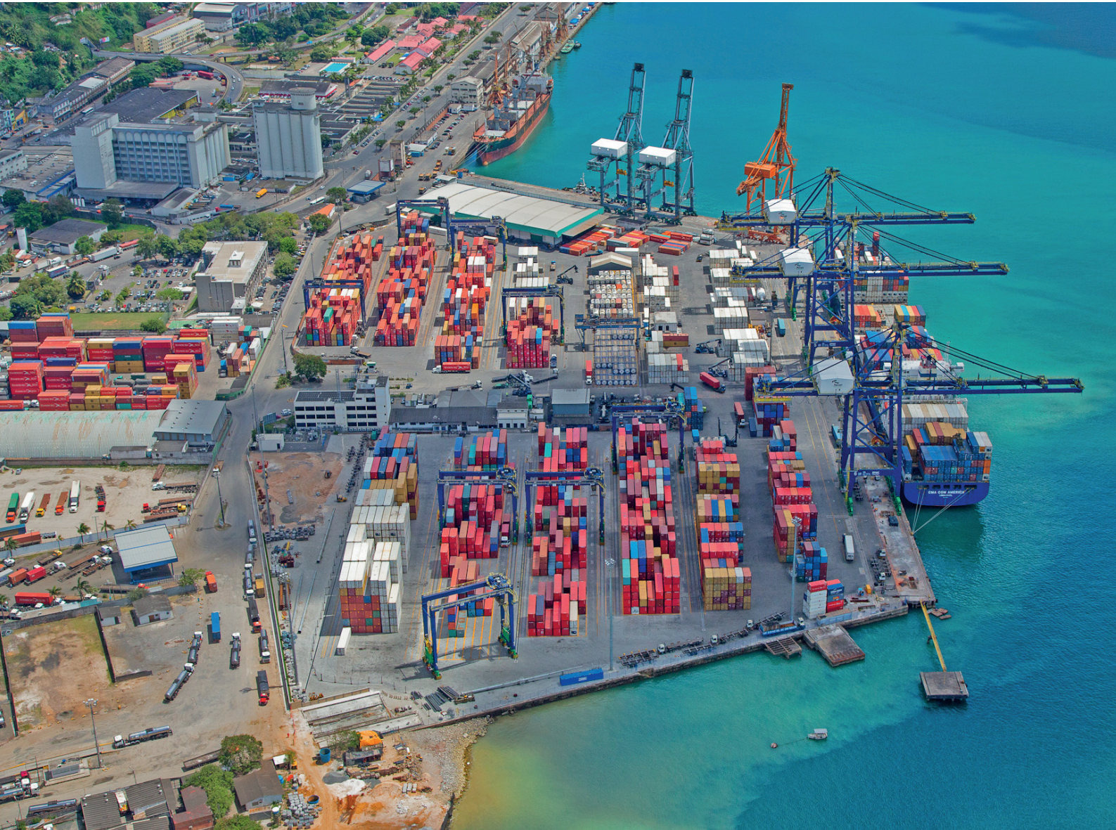
Tecon Salvador container terminal in Salvador, Bahia. Following completion of the Tecon Salvador expansion in 2012, capacity increased to 530,000 TEUs.
